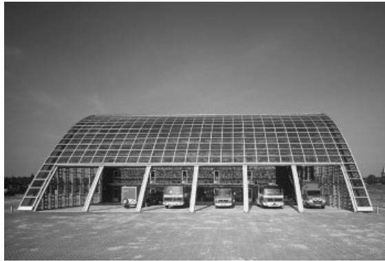
Figure 4. Fire station in Houten, Netherlands. Transparent panels have been fitted into the curved roof. Design: Philippe Samyn & Partners, Brussels, Belgium
