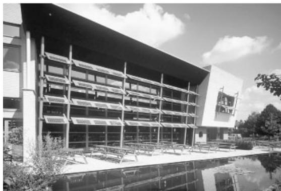
Figure 7. Façade with sun protection that includes a PV system. Fitting the integrated system of vertical blinds livens up the building and makes it visually attractive. Design: ABZ Architects, Netherlands
