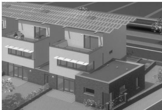
Figure 26. Zero-energy homes in Etten-Leur, Netherlands. The roofs are fitted with a steel construction that fits over the houses, so that the direction of the PV modules does not depend on the orientation of the homes. Design: BEAR Architects, Gouda, Netherlands
