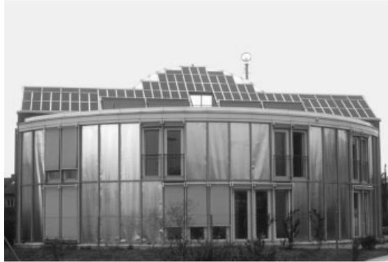
Figure 3. The Energieautarkes Haus in Freiburg, Germany, has a rounded façade that allows maximum solar entry. A semi-integrated PV system is visible on the roof
