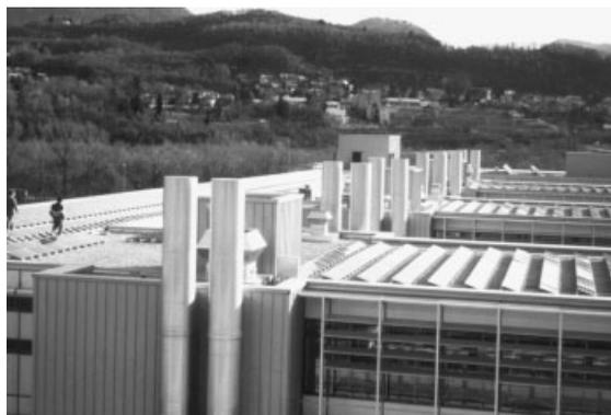
Figure 12. Roof outline of the UBS bank in Suglio, Switzerland. The detachable PV console modules form a total concept with the 'high-tech' image of the roof outline
