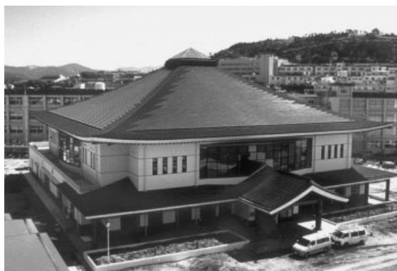
Figure 13. Houoh High School in Houoh, Japan, with a roof covering that consists of roofing tile modules. This type of PV system blends well with the traditional Japanese slate-type roof
