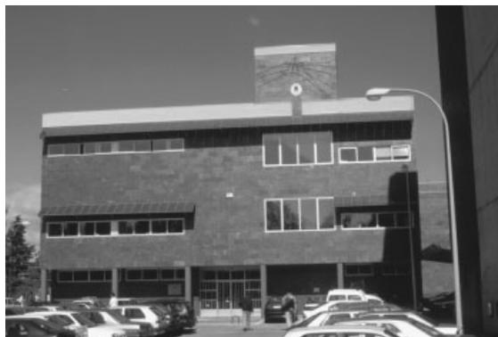
Figure 20. Solar Energy Institute at the University of Madrid, Spain. The PV system was added to the building at a later date and is also used as permanent sun protection
