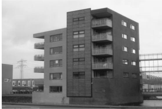
Figure 9. Apartments in the 1.3 MW project in Amersfoort Nieuwland, Netherlands. The façade consists of three blocks of colour, so that the block with blue solar panels harmonizes with the adjacent brick-coloured blocks. Design: Studio Z, Rotterdam, Netherlands
