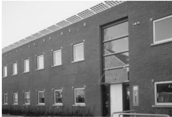
Figure 23. The edge of the roof on this office building is fitted with a glass overhang to protect the façade, which mostly consists of transparent glass modules. Design: BEAR Architects, Gouda, Netherlands
