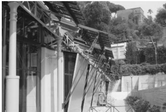
Figure 15. Children's Museum, Rome, Italy, with a PV system integrated into the sun protection that is particularly well detailed. Design: Abbate & Vigevano Architectura, Rome, Italy
