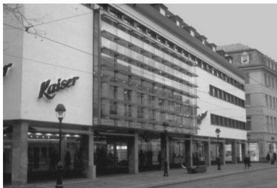
Figure 11. Modehuis Kaiser, Freiburg, Germany. A more open façade was added when the building was renovated. The huge amount of glass is protected by a glazed sun protection that includes PV cells. The system exactly fits the size and shape of the windows that it covers
