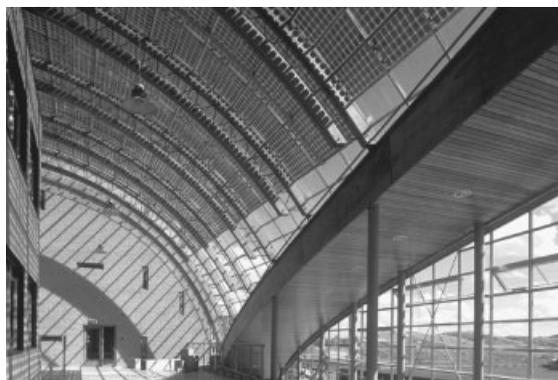
Figure 1. Interior of the conservatory in Building 42 at ECN in Petten, Netherlands, with PV system integrated into the transparent roof. Design: BEAR Architects, Gouda, Netherlands
