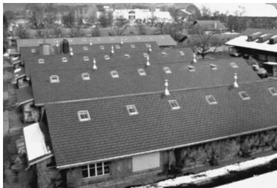
Figure 8. Horse stables in Bern, Switzerland. This historic building includes PV slates that, together with the standard roofing slates, harmonize with the old building. Colour and texture blend well together
