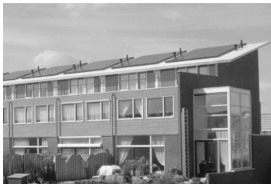
Figure 21. Homes in the 1.3 MW project in Amersfoort Nieuwland, Netherlands. The PV systems have been visibly added. The architect has accentuated this by selecting a white roofing foil. Design: Duinker & Van der Torre, Amsterdam, Netherlands
