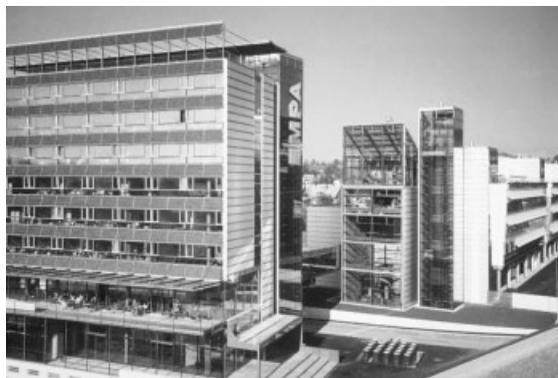
Figure 22. The Swiss Institute EMPA has integrated PV systems into the façade and combined them with movable sun protection. Design: Theo Hotz, Zürich, Switzerland
