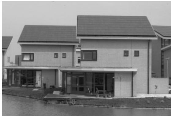
Figure 24. These houses, in the 5 MW<sub>p</sub> project in Langedijk, Netherlands, all have a large roof that is completely covered in PV modules, without drainage perforations, which emphasises the roof. Design: BEAR Architects, Gouda, Netherlands
