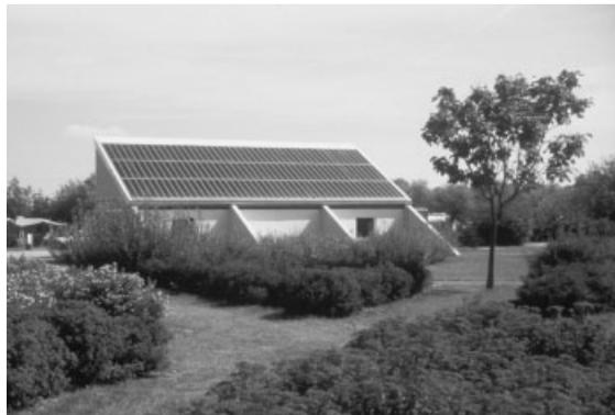
Figure 5. Toilet/shower facilities on a campsite near Poitiers, France with the PV system completely integrated into the roof
