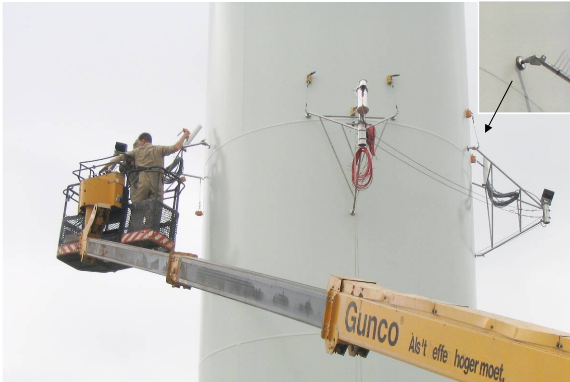
Figure 4: Installation of mounting structure with cameras, IR lamps and WLAN antennas
