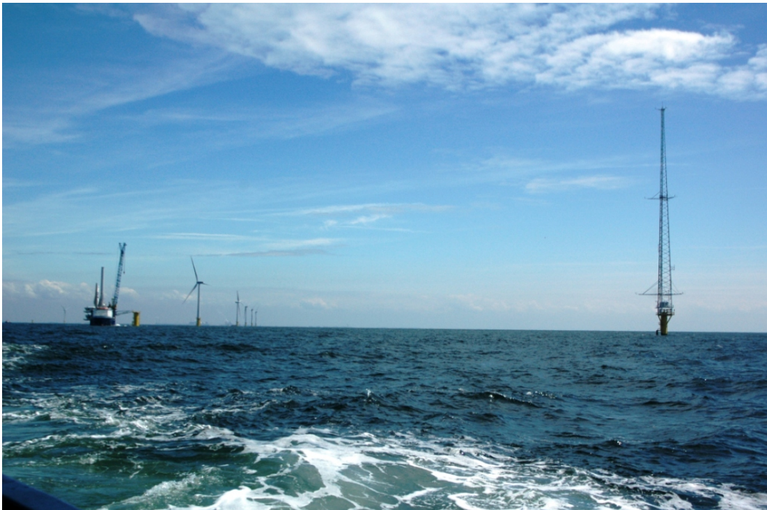
Offshore wind farm Egmond aan Zee during installation, including meteor mast near wind turbines 7 and 8. (© J. Beurskens)
