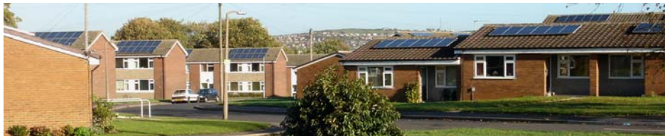
Fig. 10. Several of the PV systems installed at the Fernside Estate
