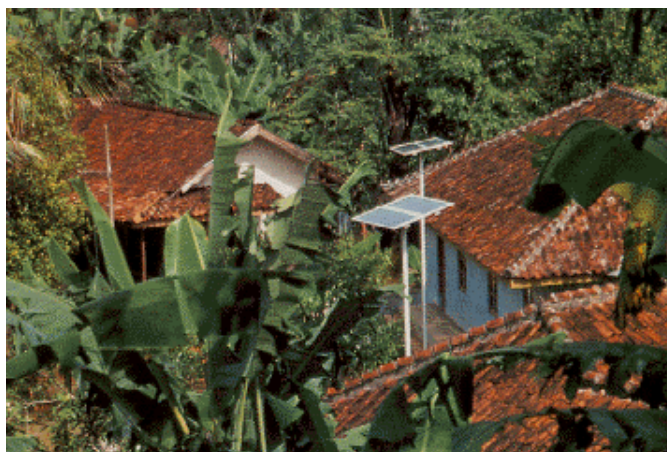
Solar Home System project in Lebak, Indonesia
